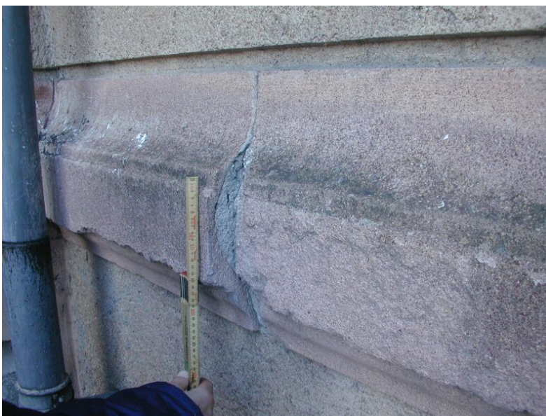
Ashlars decoration made of Portland Cement mortar. The colour is light grey and the durability is very high.
