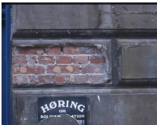
A Flaking of plaster layers
