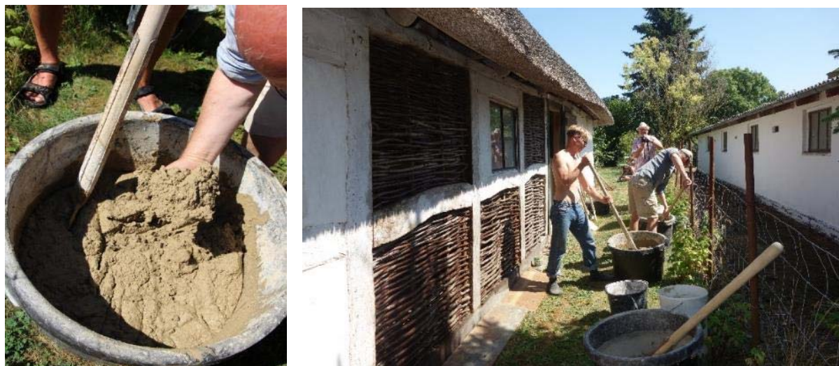
Figure 7. A tub of ready mixed clay mortar, ready for use as wattle and daub. Photo: Søren Vadstrup.
