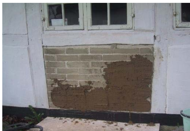
Figure 5. Repair of a fallen plaster on the adobe clay wall. Photo: Søren Vadstrup.
