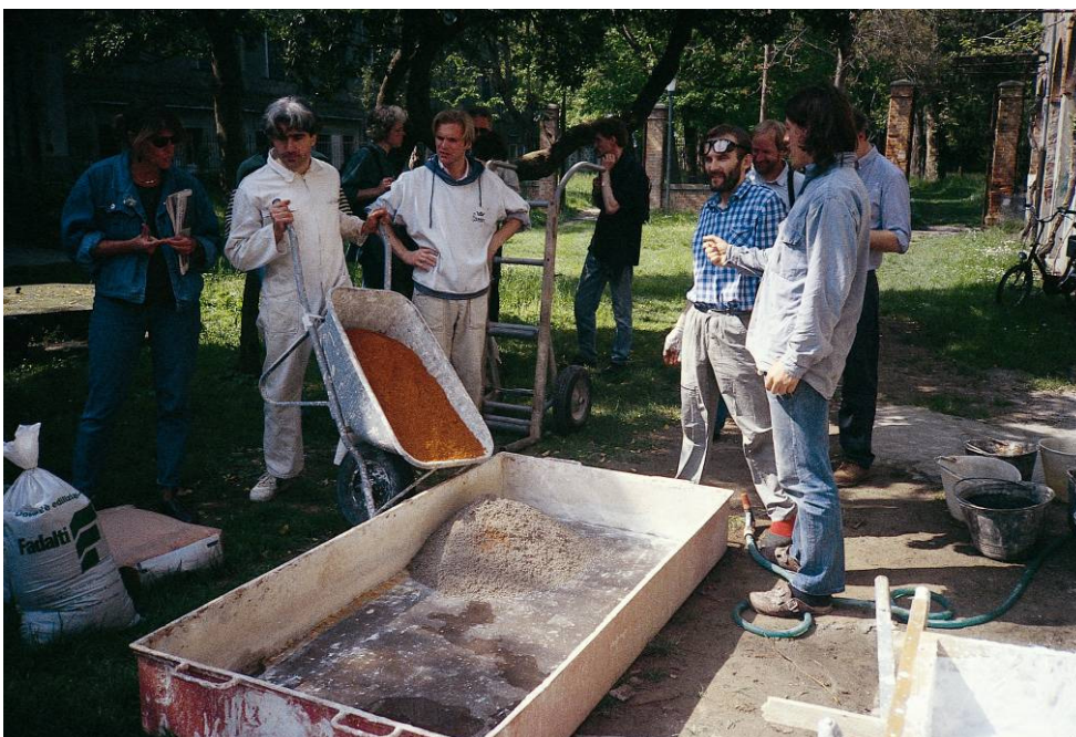
Making hydraulic mortar by putting brick dust in air lime mortar.
