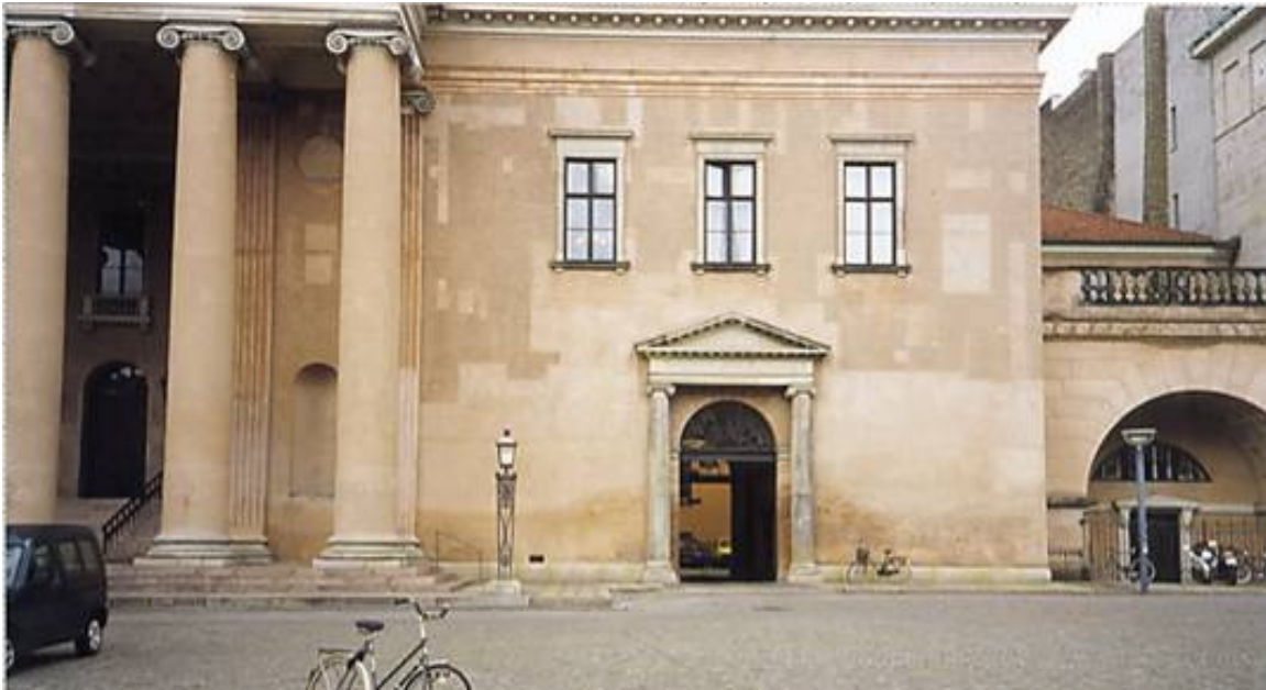
Partial repair of plaster (Domhuset, Copenhagen)
