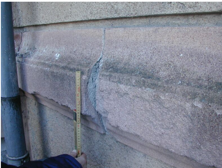
Ashlars decoration made of Portland Cement mortar. The colour is light grey and the durability is very high.
